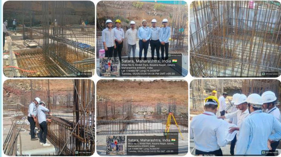
Industrial Visit for under construction Hospital Site, MVT Buildcon, Satara
